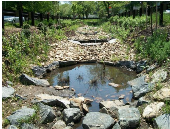
Figure 6.11 Loose Stone Check Dam
