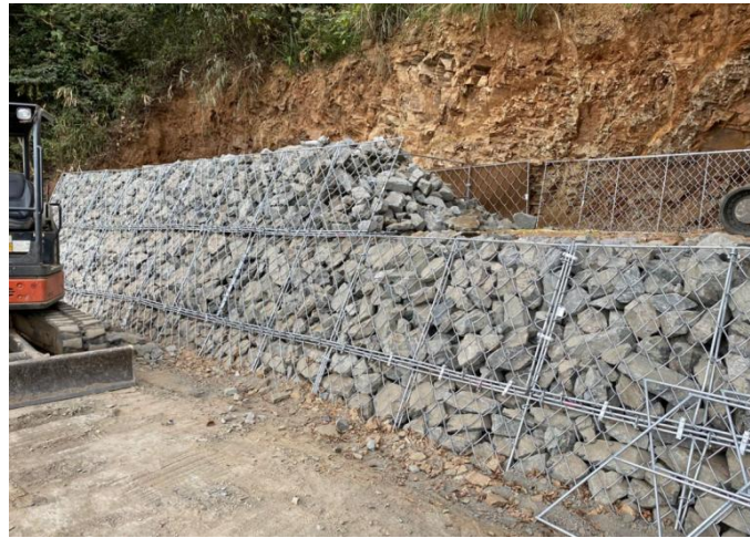
Figure 6.12 Gabion Check Dam
